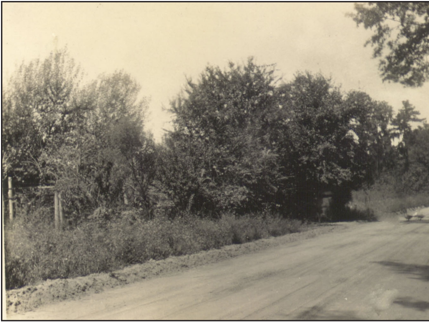
The photograph shows the State Road at the Eighteen-Mile Intersection in the early twentieth century. A notation on the photograph states that the clump of trees marks the defunct intersection of the "Road to Dorchester." William Henry Johnson (1871-1934) produced the photograph. The image is in the William Henry Johnson Scrapbook, circa 1920-1923, among the photographic collections of the South Carolina Historical Society in Charleston.
