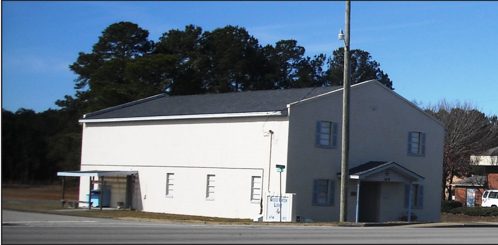
The Goose Creek Masonic Lodge stands near the eighteen-mile intersection on St. James Avenue in 2014. There, the Eighteen-Mile House Tavern once served as a threshold to the Carolina frontier and as the cradle of the Deep South.
